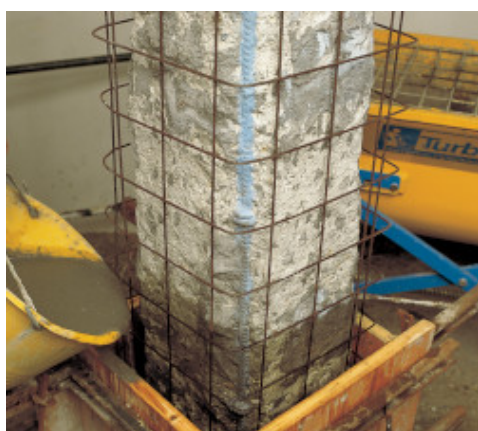
Turnarea in cofrag
